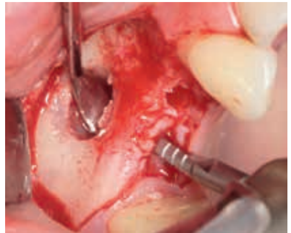
Fig. 5 Mechanical preparation of the implant cavities.
